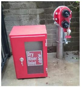
A dry riser is a system of pipe work and valves that runs up through a building. The system allows fire fighters to easily access water at a high pressure from each floor of the building. In normal circumstances these systems sit unused and can become damaged, neglected or even vandalised.
